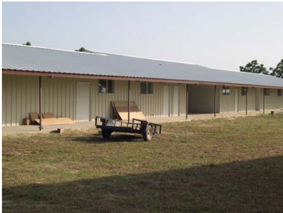
The main clinic building is completed, ready for cleaning and all medical equipment installation.
